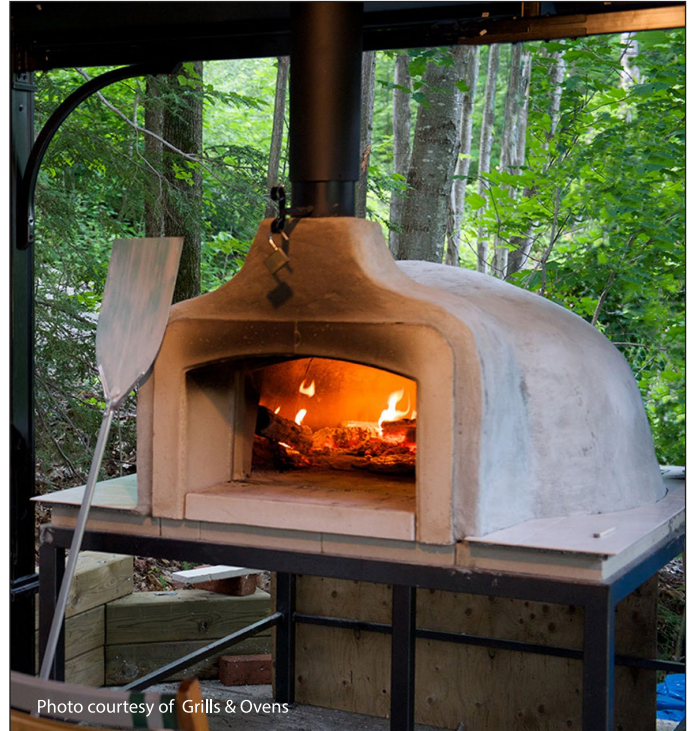
This traditional wood-fired pizza/bread oven uses perlite as an insulator to hold and stabilize the heat.
